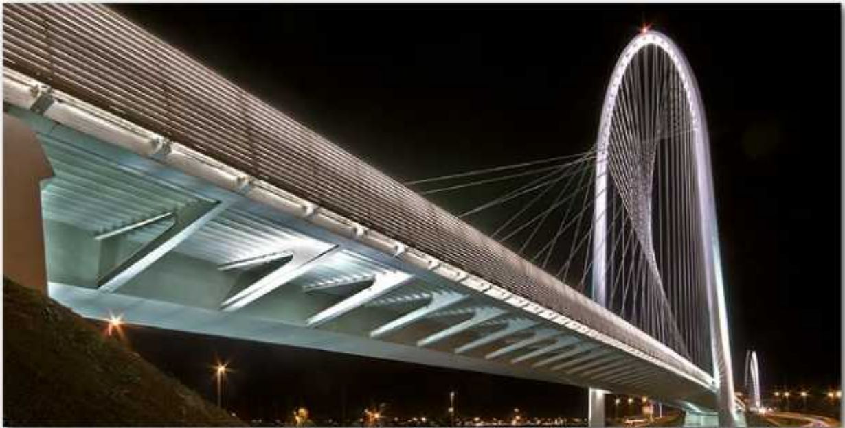
Calatrava bridge (Italy) - Luxsolar 2013 MIOL AB (White light day/twilight mode - Red light night mode)
